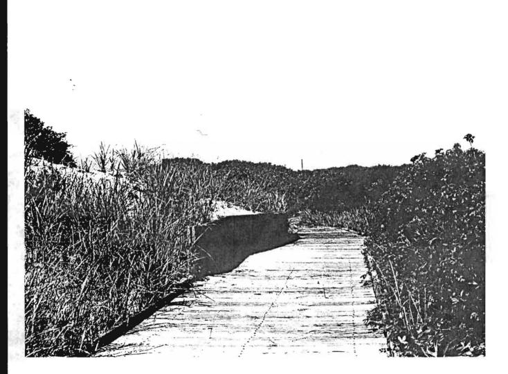
Figure 3 - Planked walkways help to ensure that neighboring vegetation will not be trampled by pedestrians.
