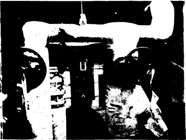
PIPES FEEDING DORMITORY HEAT EXCHANGER UNITS have recently had to be dismantled to remove the exchanger units for repairs.
