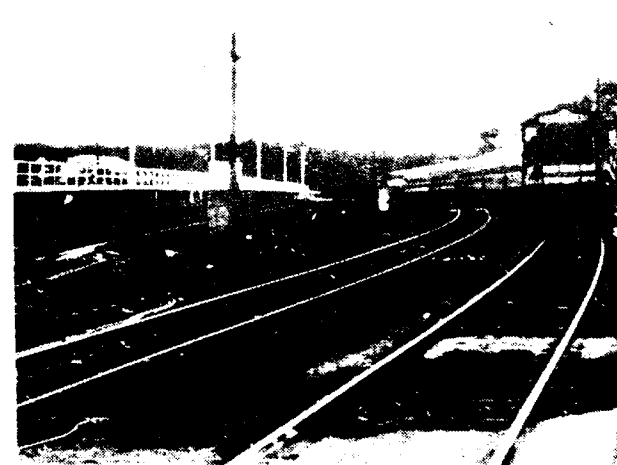
Stony Brook train station after.
