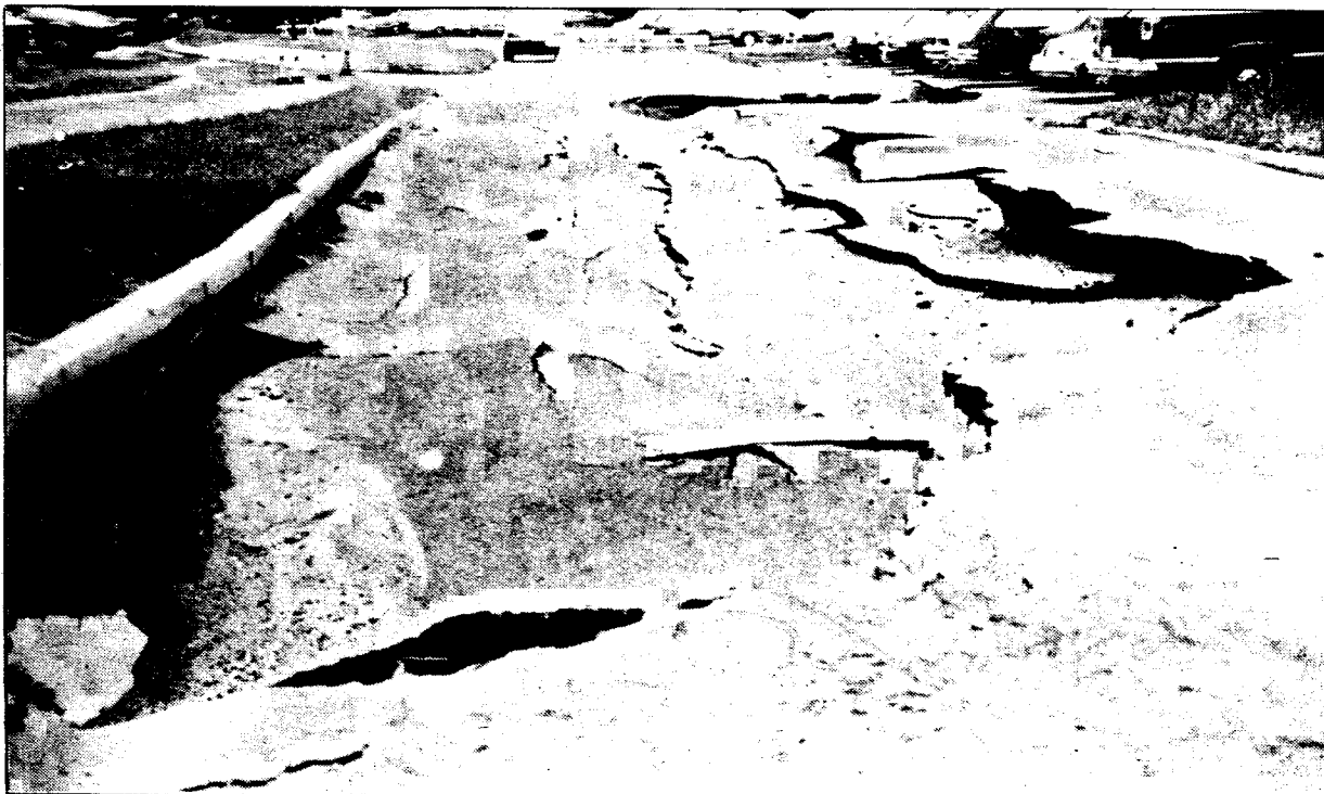
Statesman / JoMarie Fecci A roadway in Roth Quad, undercut by a broken water main, collapses and strands residents' cars in the parking lot.
