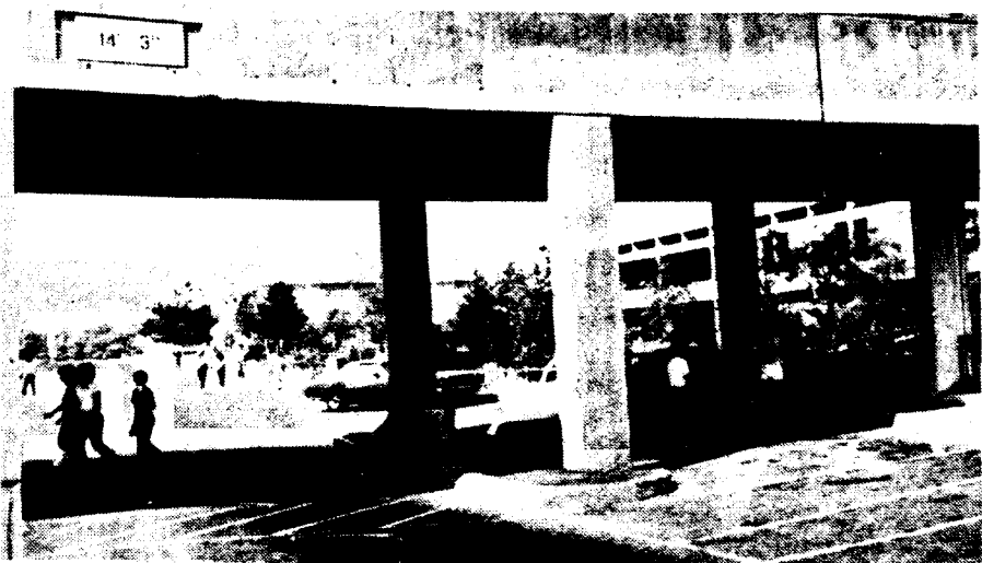
The Bridge to Nowhere at the State University at Stony Brook.
