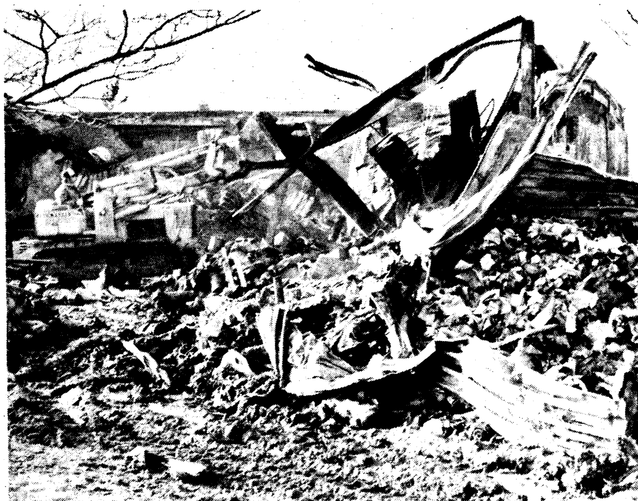
Rubble from a fire that burned for 15 hours last week and destroyed most of the Commissary.
