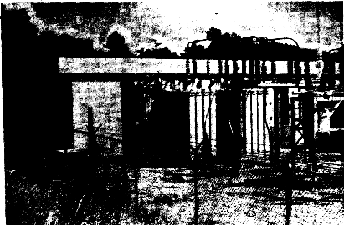
ONE OF THE SUBSTATIONS of the Physical Plant which Physical Plant Director Kevin Jones said operated properly during the blackout
