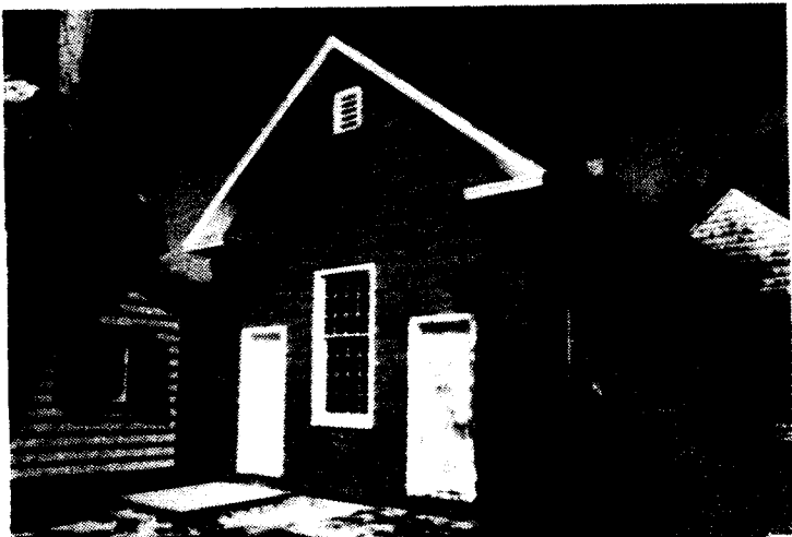
A view of the 19th century schoolhouse, another feature of The Museums at Stony Brook.
