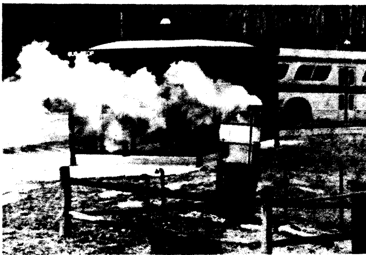
STEAM ESCAPES from a manhole cover near the Tabler Quad steps due to a broken pipe. Statesman/David Jasse
