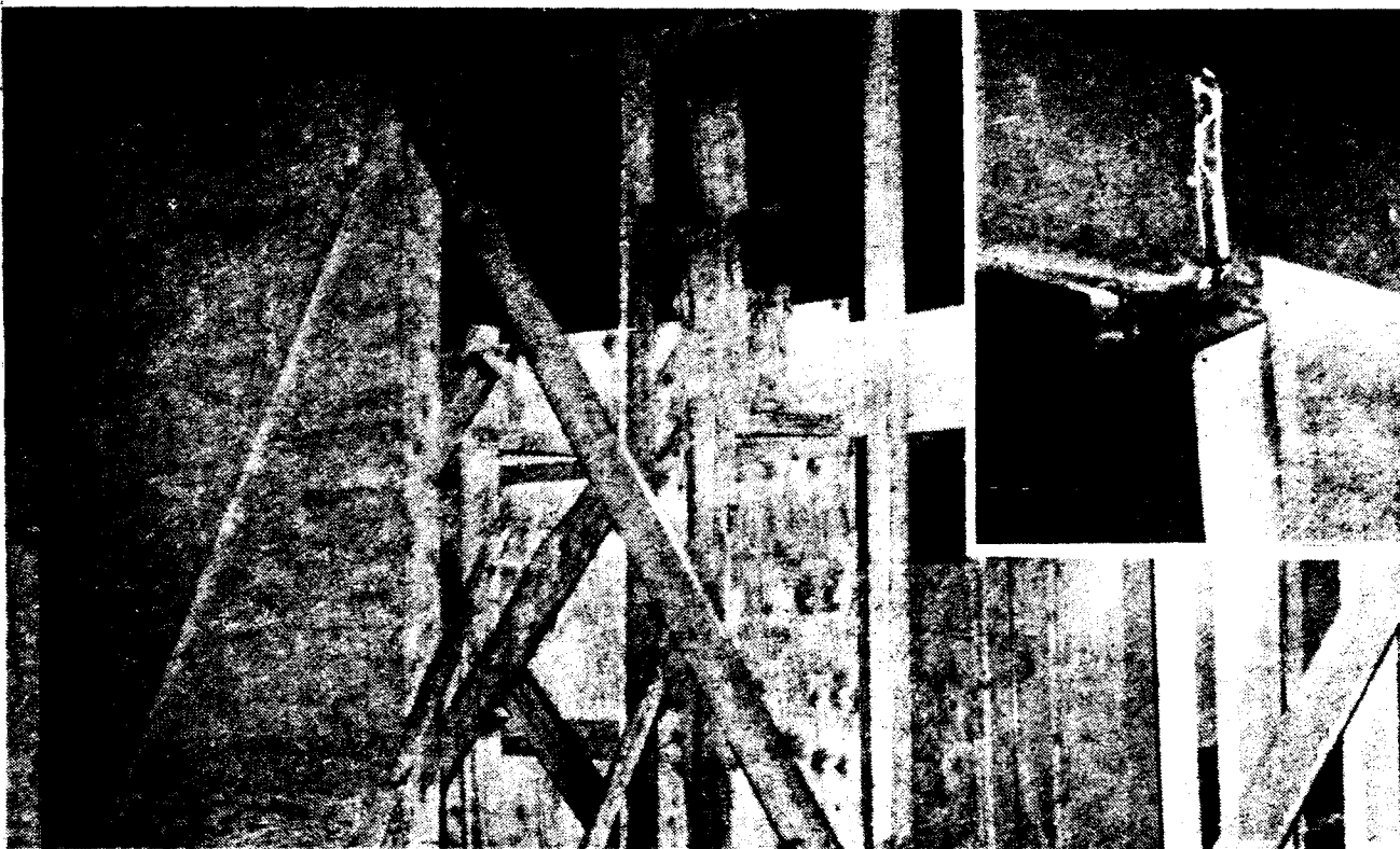
TIMBER: Wooden supports erected to hold a cracked beam (inset) at the school of Allied Health Professions in the Health Sciences Center
