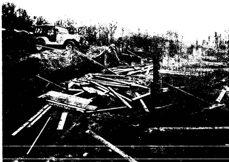
NEED A PLACE TO SETTLE DOWN? Behind Kelly C and D, the University is expanding a siting basin for campus drainage. The spillway, pictured here, will, upon completion, separate ponds in which silt and other small particles settle to the bottom and are filtered out of the water.
