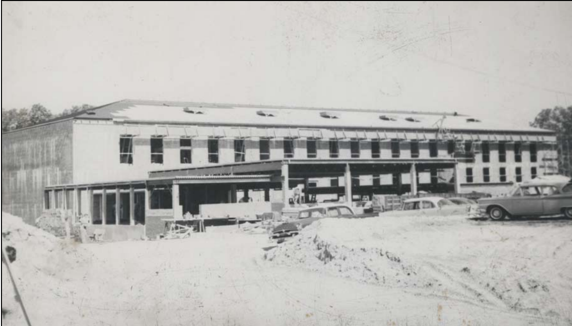
Stony Brook: The “New” Chemistry building under construction.
