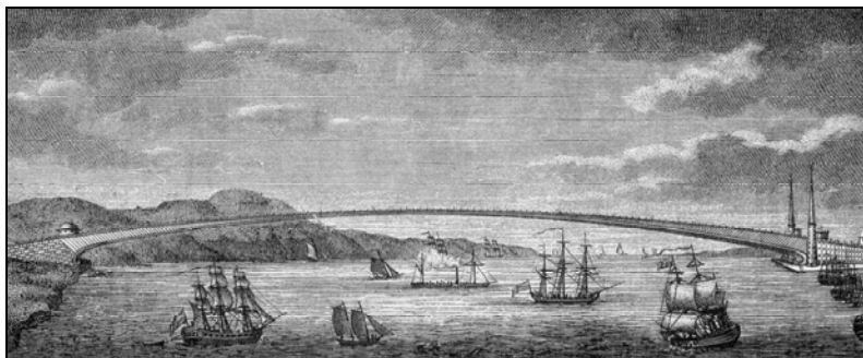
View of Pope's Flying Lever Bridge, 1811.
