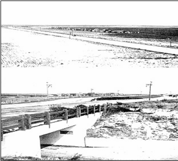
Example of the hydraulic fill along Oceanview Parkway, Jones Beach Barrier Island, 1938.
