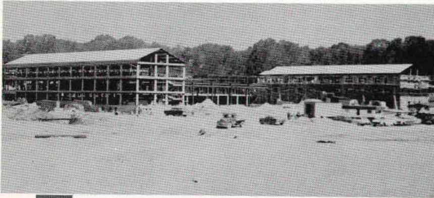
Stony Brook construction ahead of schedule . . . miracles never cease.
