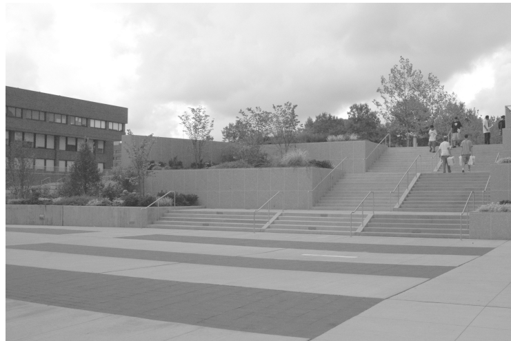
STALLER PLAZA: BEWARE OF SPRINKLERS, Courtesy of Jowy Romano
