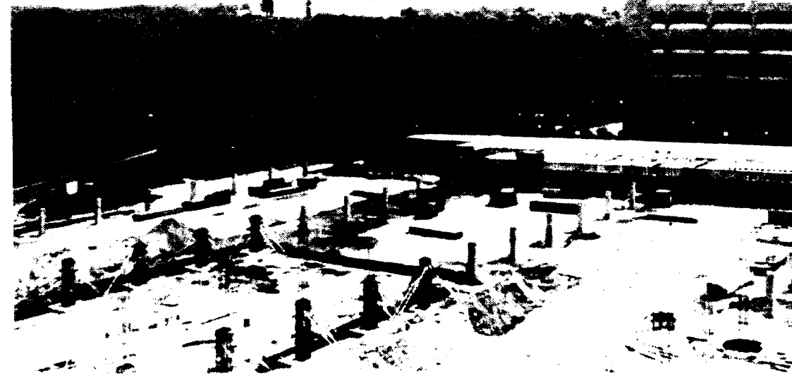
CONSTRUCTION AT THE Administration parking lot caused protests yesterday at G- and H-Quads.
