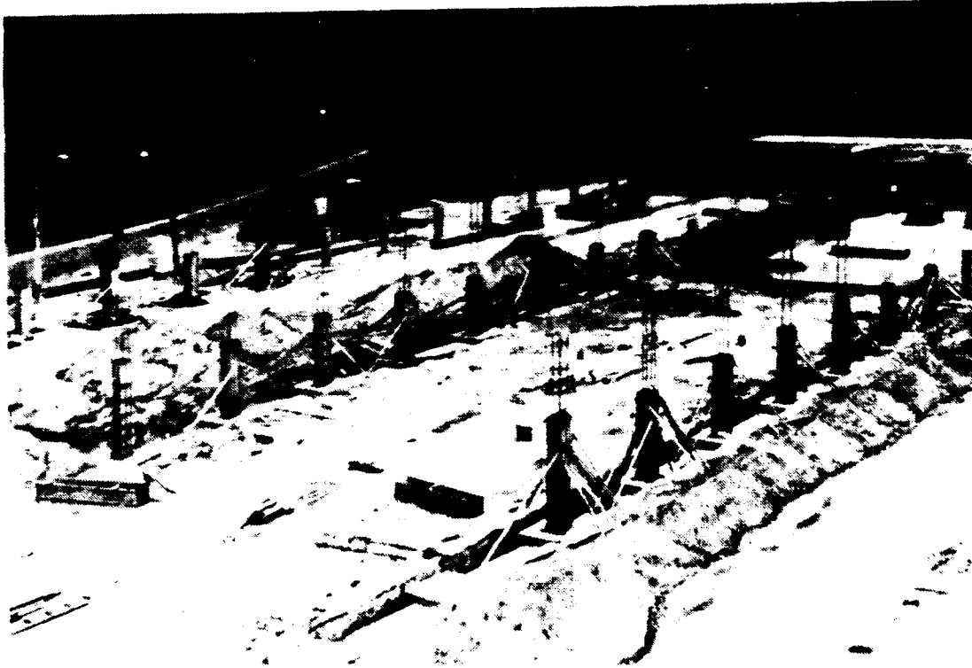
THE ADMINISTRATION PARKING GARAGE under construction in September. This resulted in a reduction of spaces in G and H Quad lots for resident students.
