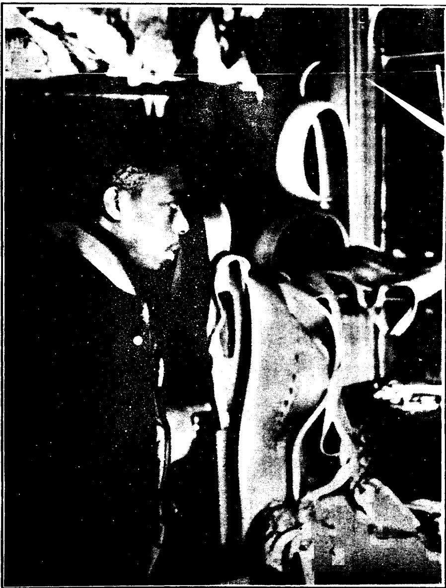
Resident assistant Sedgewick Jeanite surveys damage to Dreiser room next door to dorm charred by fire last Tuesday
