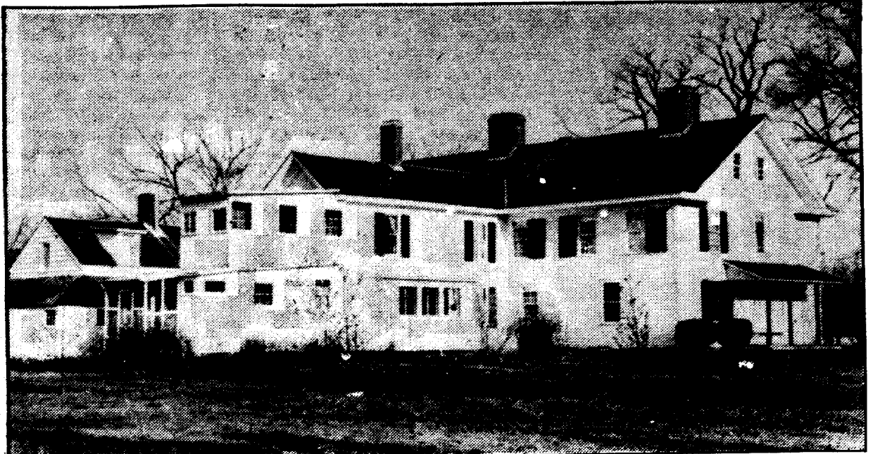
Cornelia Floyd Nichols enlarged the northwest wing of the Floyd Estate (left) in the 1920s. It was the last addition to the house.
