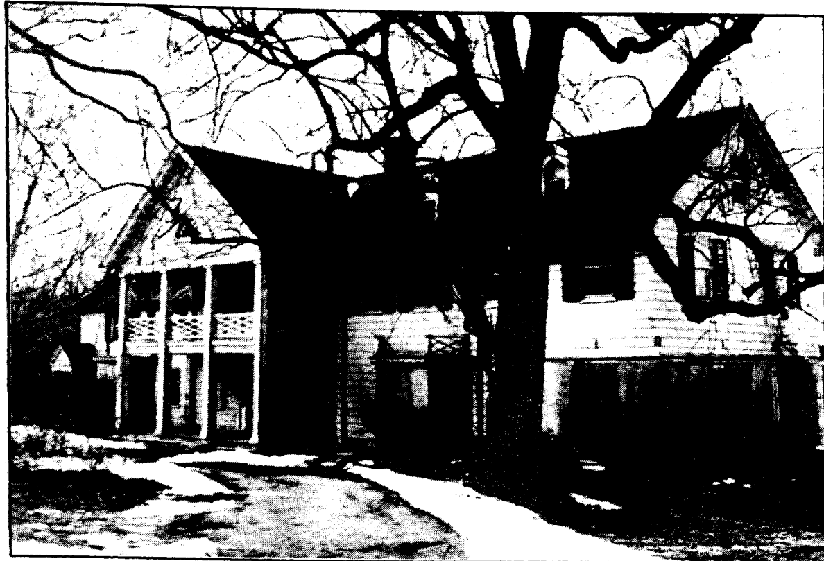
The deteriorating Childs Mansion in Crane Neck.
