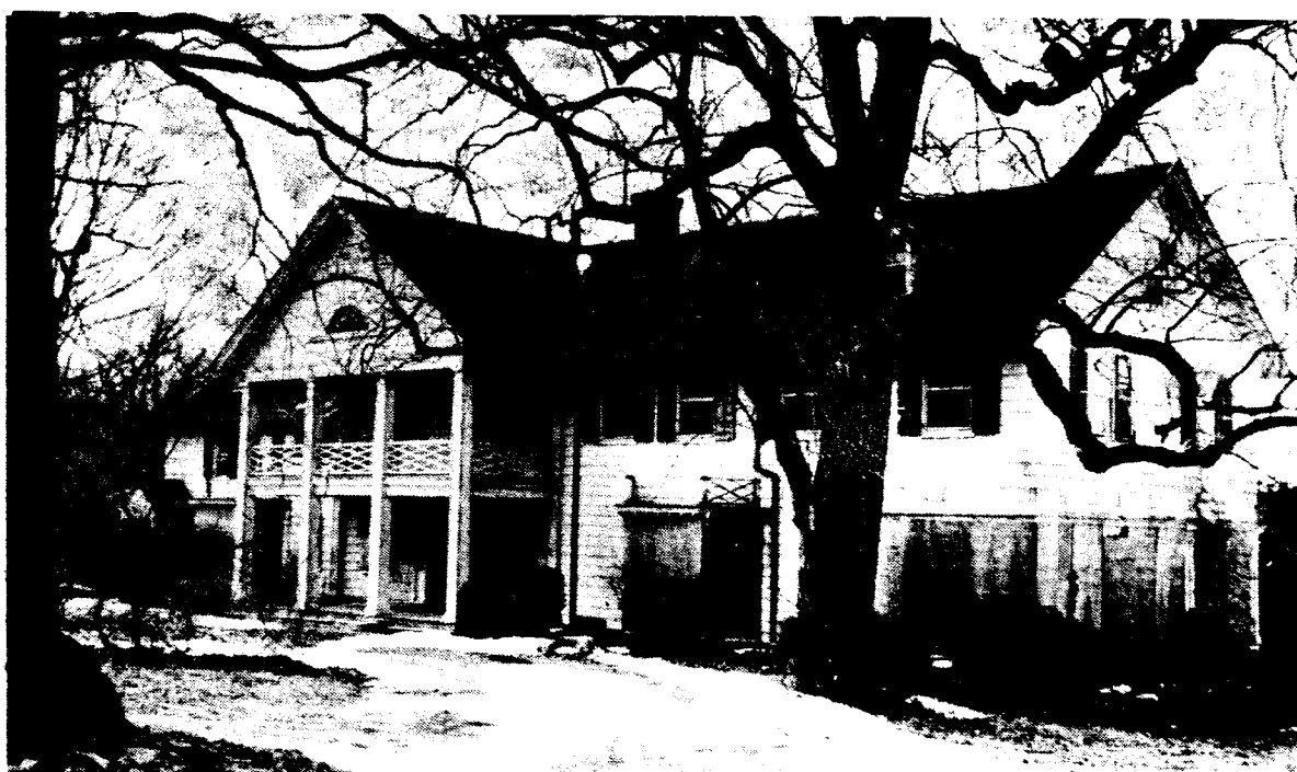
The deteriorating Child's Mansion whose future is still in limbo.
