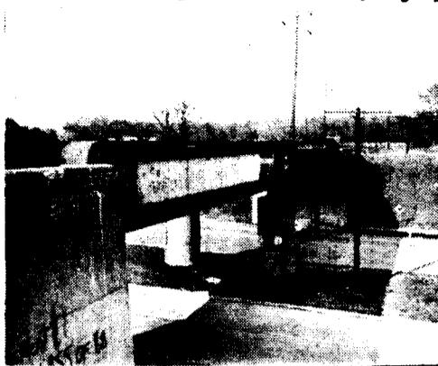
The Stony Brook railroad trestle bears the marks of the nearby university.
