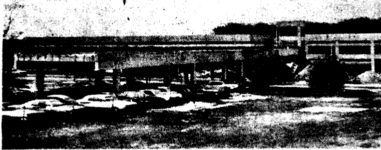
The campus center bridge: a new concept in outdoor art shows.
