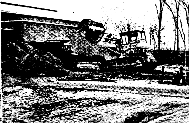
TUNNEL TO NOWHERE: Workmen are building a tunnel to connect buildings for utility purposes. photo by Mike Amico
