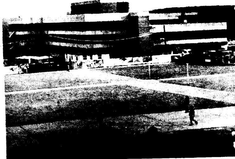
1st ANNIVERSARY: The Administration Building, which was started a year ago this week, is expected to be open in time for the start of the Fall semester.
