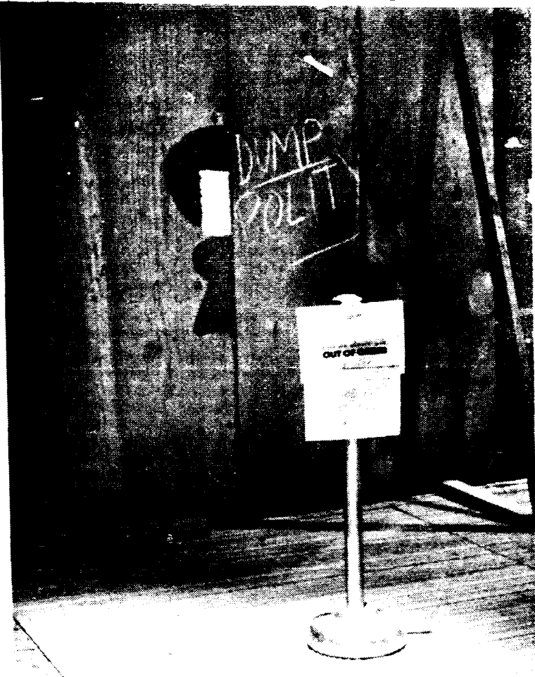
BROKEN: Glass doors, which were the main entrances to the Union building, are now boarded up. There has been considerable damage to many of the areas of the building, and I.D. checks have been instituted to alleviate the problem of building security.
