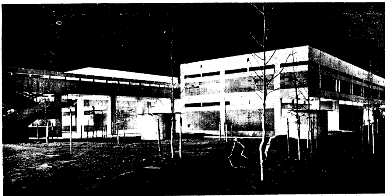
UNION BUILDING: An escaped inmate was apprehended here Wednesday night after having annoyed students on campus for at least two days.
