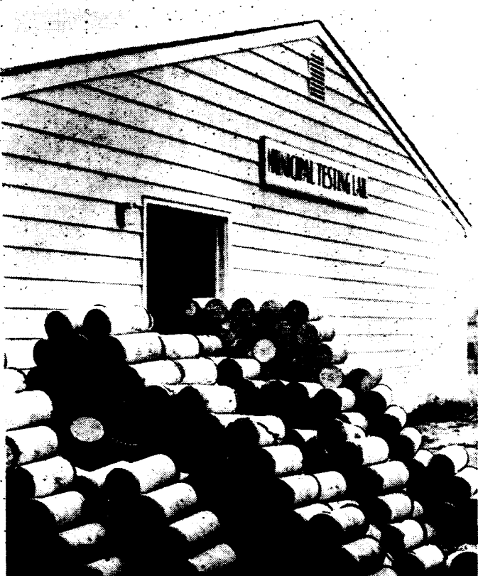
Students driving from Kelly to the student union may have noticed a small wood frame structure bearing the designation "Municipal Testing Lab." According to Charles Wagner, Director of Facilities Planning, it houses equipment for testing the quality and strength of concrete used in campus construction projects, in order to make sure that builders are living up to their contracts. The cylindrical objects shown above are dated samples of concrete waiting to be tested. The laboratory is one of three such buildings being used by the State University Construction Fund for offices and testing facilities.
