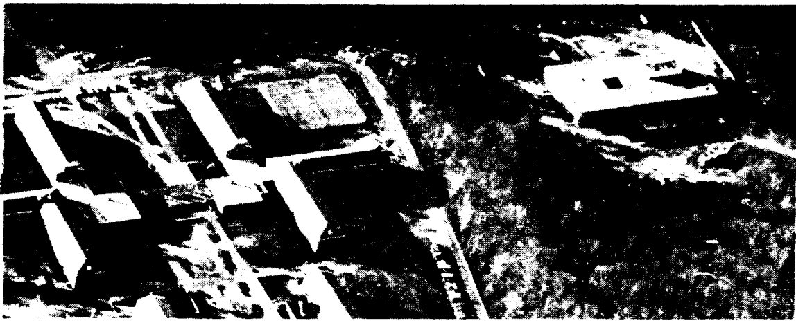
NEARING COMPLETION: The Marine Regional Headquarters and Laboratory building, north of H quad in this aerial view, will conduct tests on the surrounding environment. photo by Bob Weisenfeld
