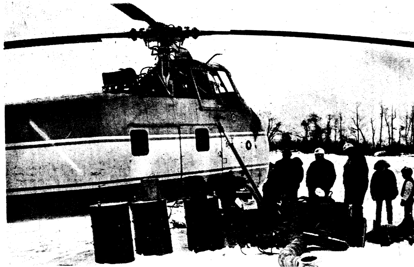
Before picking up ducts, helicopter readies flight equipment and fuels up.
