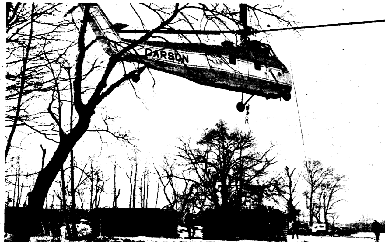
Cables from helicopter are fastened to air ducts.
