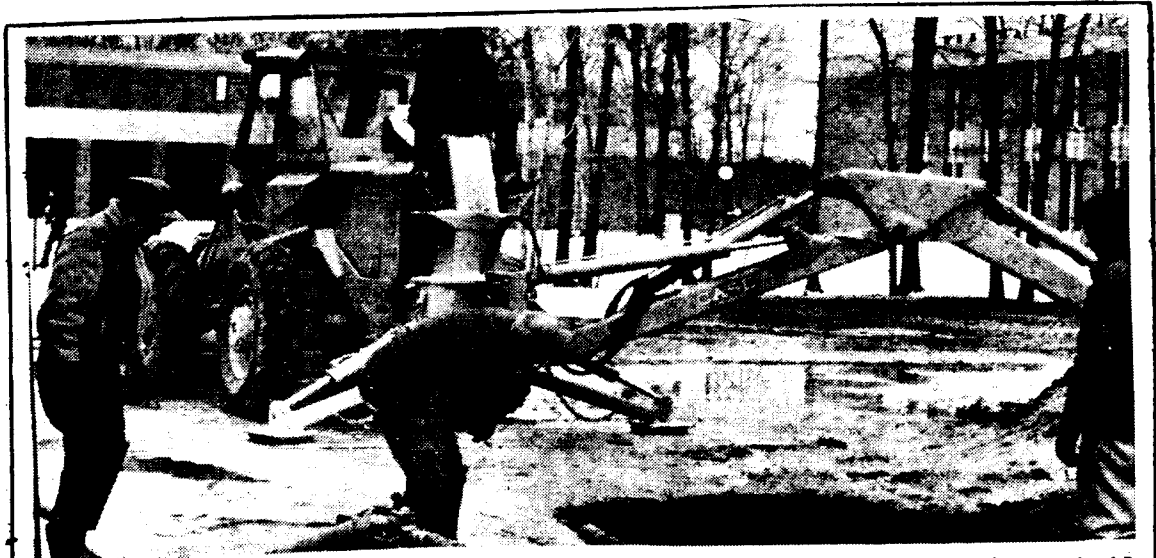
BROKEN WATER MAIN: Students living in Roth Quad were without running water for nearly 12 hours yesterday when a 10 inch supply pipe broke under the grounds surrounding the Engineering Buildings. The breakage, reported to Security early Monday morning, was repaired (above) yesterday afternoon by workers of the university's plumbing shop along with Maintenance Director Clifford Decker. Maintenance officials believe the clean break in the water main was caused from the weight of shifting clay, made heavier by soaking rain and snow, lying above it. photo by John Sarzynski
