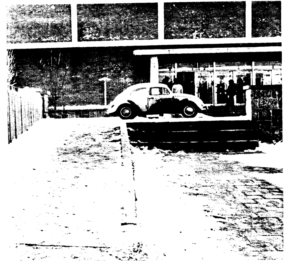
SNOW COVERED RAMP: Although there is a ramp between the Student Union Building and the Gym, the icy layer covering it makes it more of a hindrance than a help to the handicapped. photo by Larry Rubin
