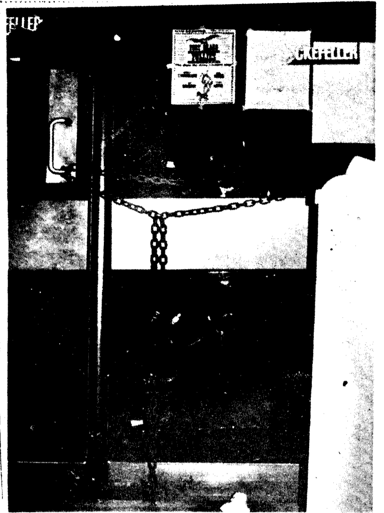
CHAINED DOORWAY: At back entrance enhances exterior appearance of the union.
