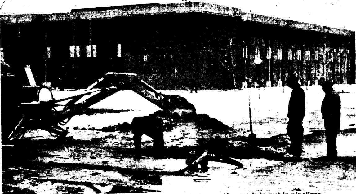
UNDERGROUND: Construction workers have been digging up the roads to put in pipelines. photo by John Sarzynski
