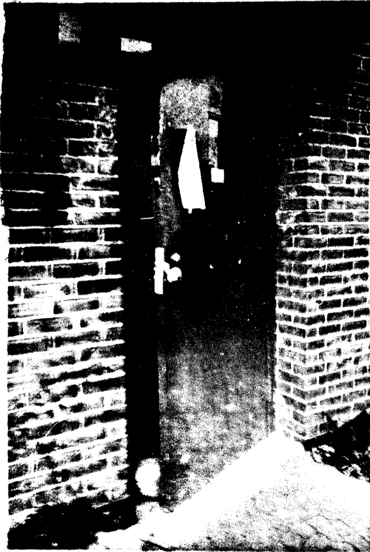
SPEEDY REPAIRS: Early last semester, this entrance to Gray (left), lost its doorknob. It was promptly repaired in a scant four months. A week later it was broken again — and has been that way ever since.
