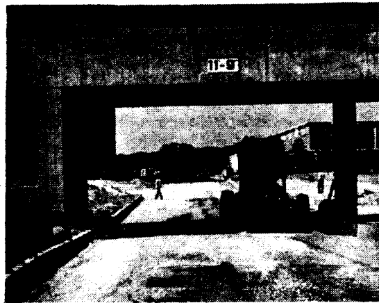
UNION BRIDGE: The clearance sign will have to be changed as the road under it was lowered over two feet.
