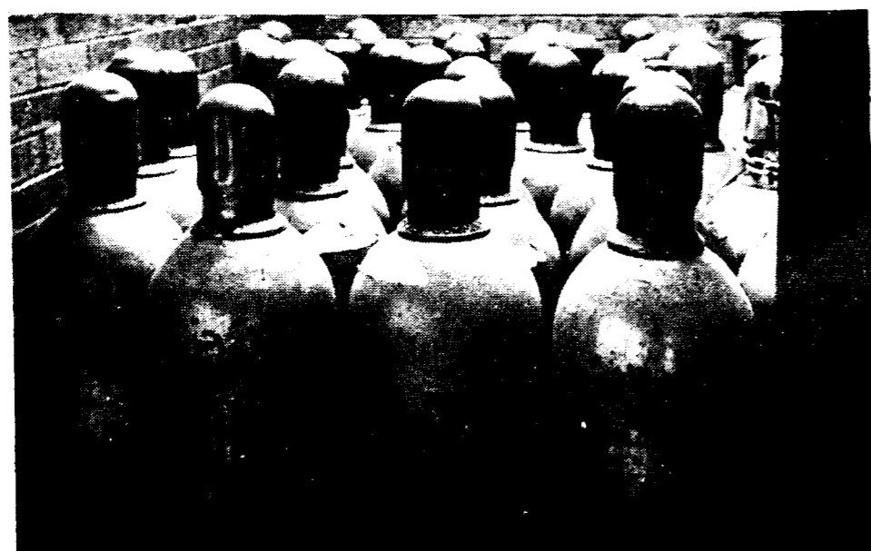
The "torpedo room" houses oxygen cylinders and is part of a volatile chemical shed. Statesman's tour guides joked that the lack of a skylight often causes the cylinders to freeze together when it rains.
