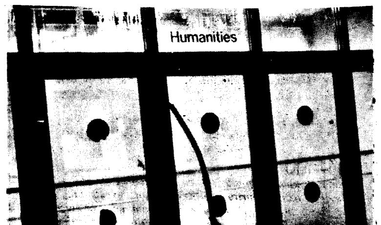
A HOT WATER PIPE BURST and flooded the entrance of the Humanities building late last night.
