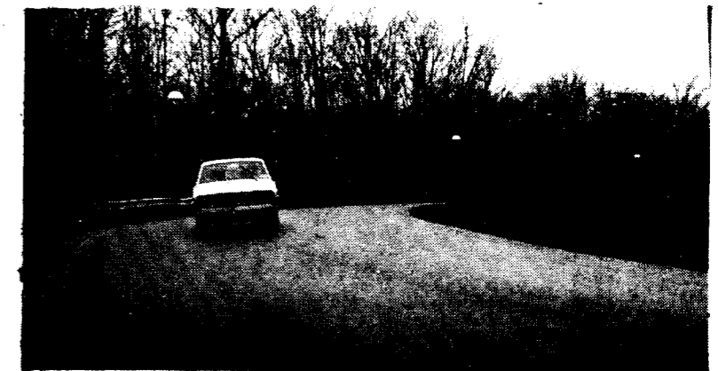
"DEAD MAN'S CURVE" behind the Graduate Biology building is banked the wrong way and has been cited by many students as a safety hazard.
