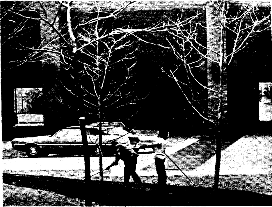
Contractor's crews planted sod behind the new Graduate Chemistry building last week, giving an early start to Clean and Green Days as they finished exterior site work on the new facility.
