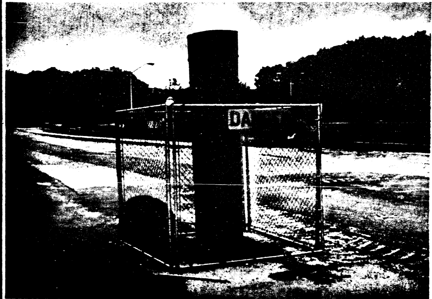
The manhole in the Light Engineering parking lot into which Raftenberg fell is now enclosed. However, one hour before the accident occurred, Security was aware that the cover was not in place. The parents are suing the State for $3,000,000 for negligence.
