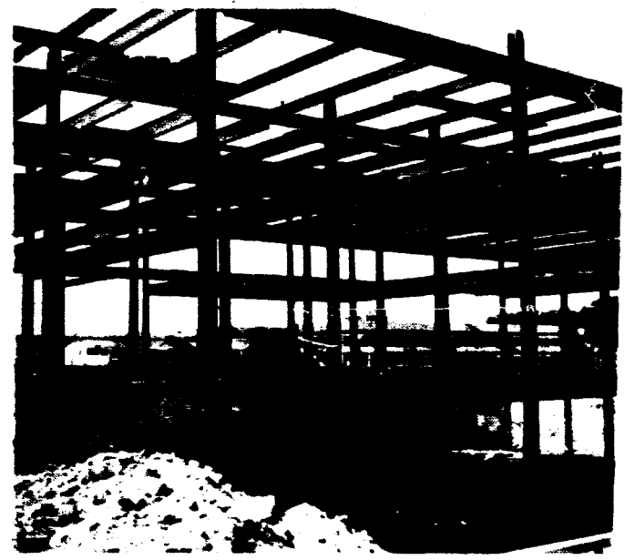
OPENING LATER: Construction on the Fine arts complex will complete Phase one in 1974.
