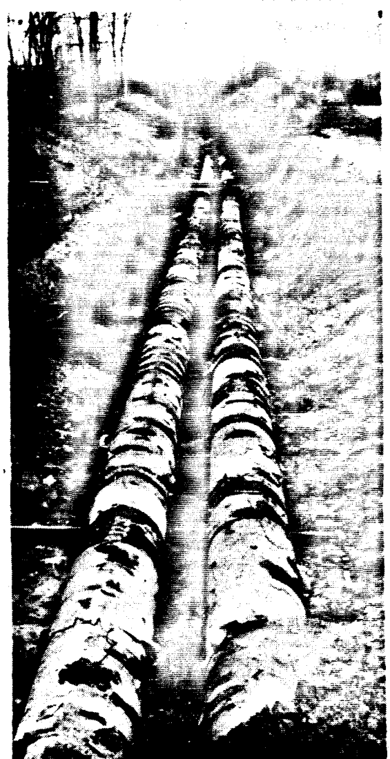
Statesman photo by Al Tarigo THE INSTALLATION OF THE HIGH-TEMPERATURE HOT-WATER HEATING SYSTEM on Loop Road between Stage XII and Roth Quad is scheduled to be completed and the road reopened by the middle of March if weather permits, according to a University spokesman. However, construction will continue in Stage XII and Roth through the summer as workmen continue the installation of the system into those Quads. The entire project is scheduled to be complete by August.
