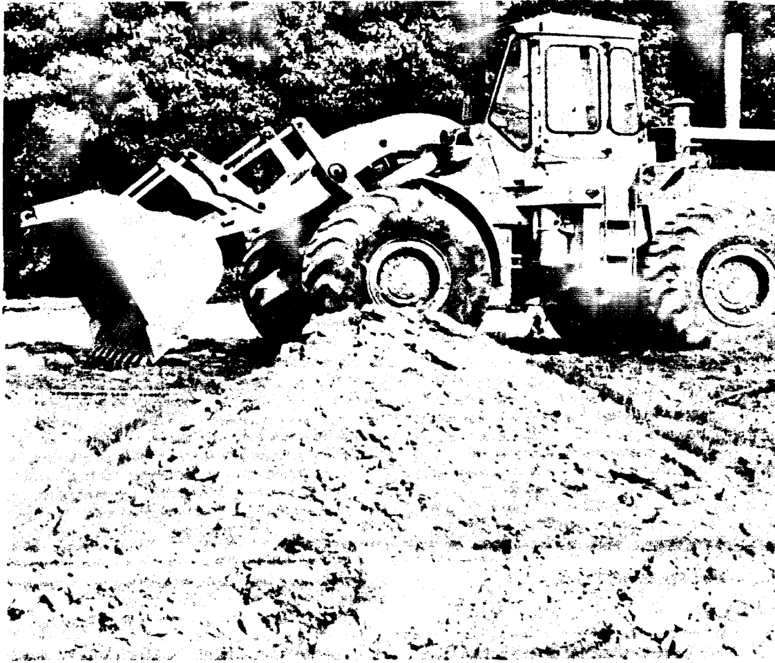
CONSTRUCTION IS UNDERWAY ON THE SOCIAL AND BEHAVIORAL SCIENCES BUILDING, which will be located adjacent to the Lecture Center, the Humanities Building and the current social sciences complex. It is cited for completion in 1978.
