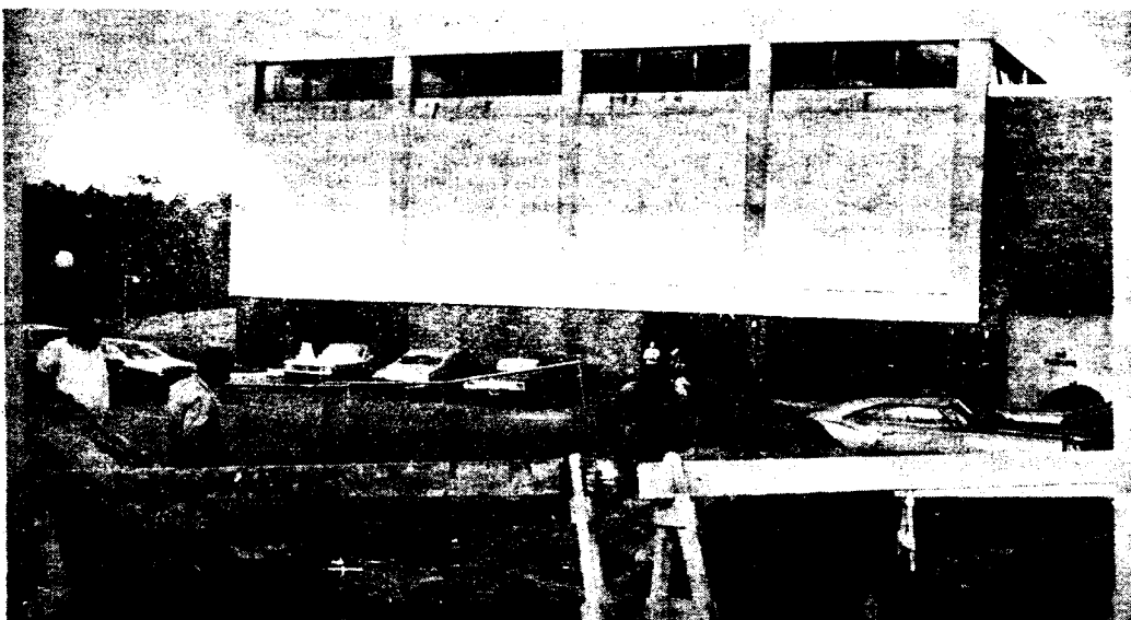
THE PHYSICAL PLANT now houses a new boiler which could alleviate the campus heating problem.
