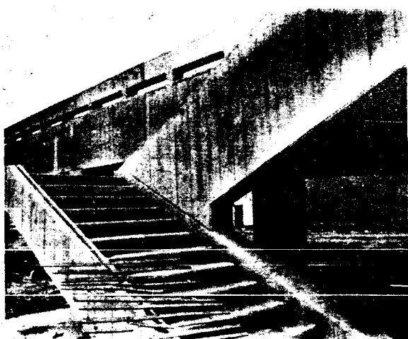
THE BRIDGE TO NOWHERE was dedicated last Friday — but it was not complete, a staircase handrail was and still is missing.
