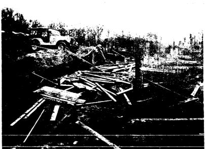
NEED A PLACE TO SETTLE DOWN? Behind Kelly C and D, the University is expending a silting basin for campus drainage. The spillway, pictured here, will, upon completion, separate ponds in which silt and other small particles settle to the bottom and are filtered out of the water.
