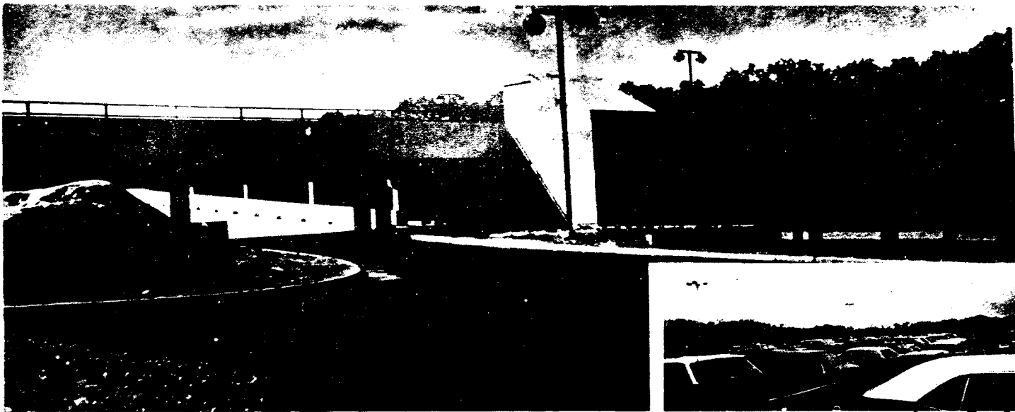
THE NEW PARKING GARAGE in the Health Science Center, scheduled to open next month will not relieve this campus's parking crunch and filled parking lots (inset) will still be common. Statesman/Karen Bales
