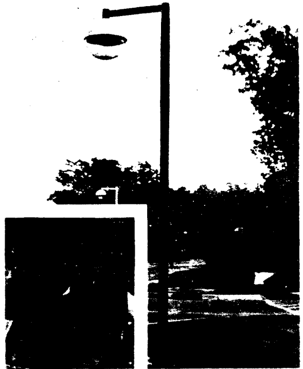
POTENTIAL SAFETY HAZARD is what Director of Environmental Health and Safety George Marshall called this light pole at the entrance to the Tabler parking lot. A block of wood (inset) was inserted to stop the rocking of the pole.
