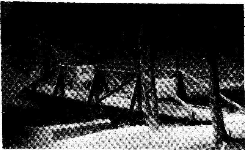
The bridge built over the other stony brook.
