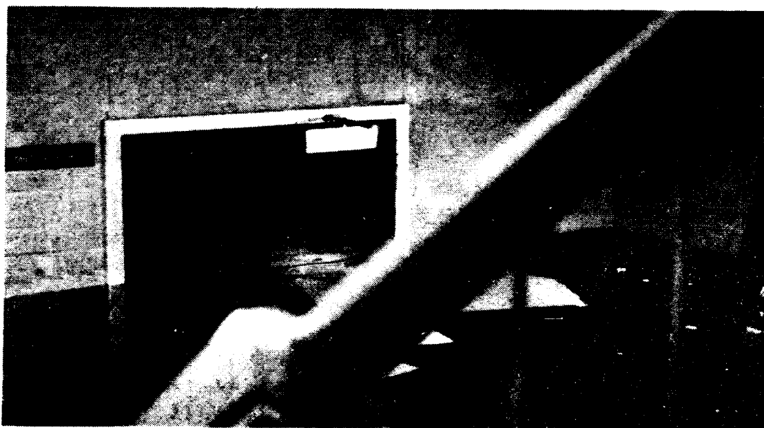
THE DOOR to a dressing room in the basement of the Fine Arts Center almost covered by water
