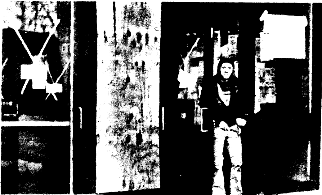
IN ADDITION TO BEING A FIRE HAZARD, broken doors make access to and exiting from the Stony Brook Union a difficult task.
